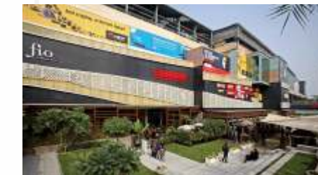
South Bridge - Nehru Place, New Delhi
