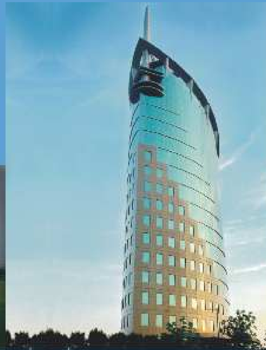
Gateway Tower, Gurgaon
