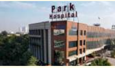
PARK HOSPITAL, MOHALI
