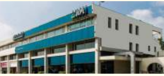
JLL INDUSTRIAL AREA
