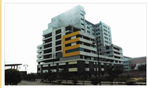
'TDI Business Centre' nearing completion
