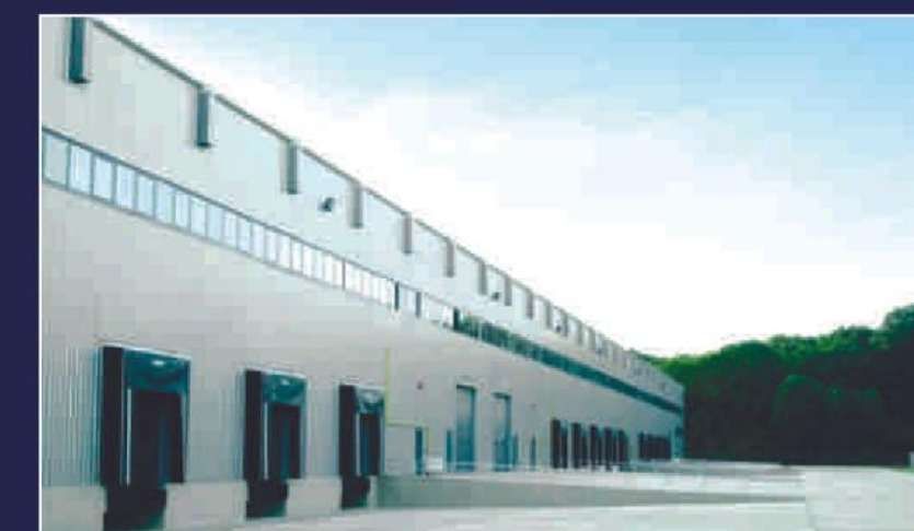
GOYAL BUILDER LOGISTIC PARK - BANUR - TEPLA ROAD
